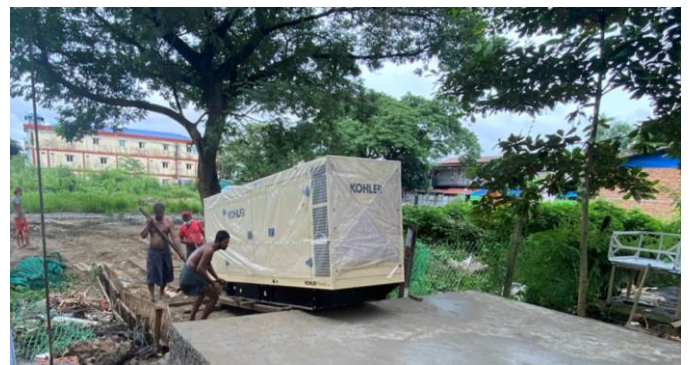
A 2,558 kilo generator put in place 'by hand' (!)
